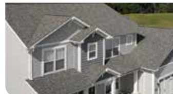
ROOFING AND VENTILATION
