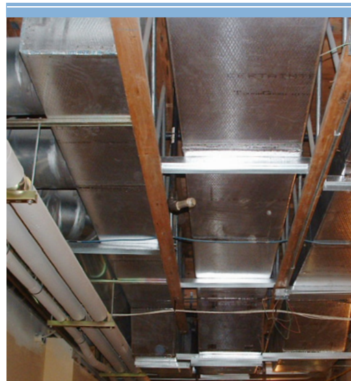
Installation of fiber glass duct board
